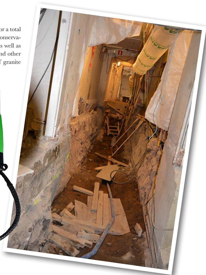
“Because of the limited space, the boulders have to be manually removed. So there is plenty of holes to be drilled”, says Jyrki Metso.
