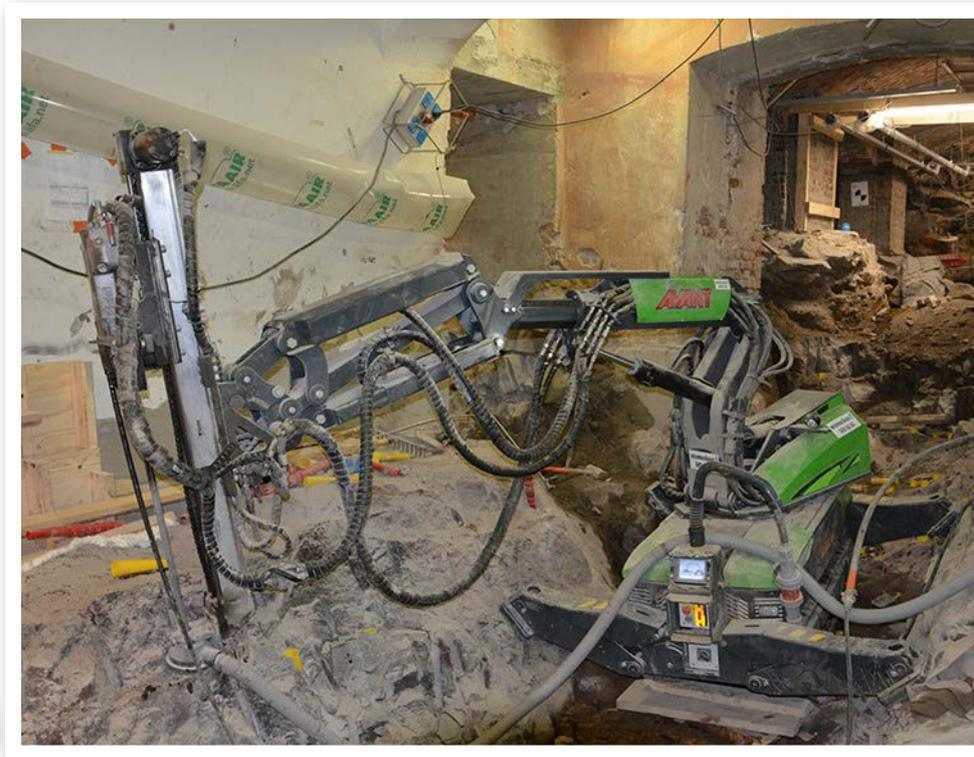
The renovation started last November and will last for a total of two years. In addition to a thorough interior conservation, the first floor is expanded for extra rooms as well as space for heating, ventilation, air conditioning and other building service equipment. The first floor stands on top of granite bedrock, which requires 500 m<sup>3</sup> of rock to be removed.
